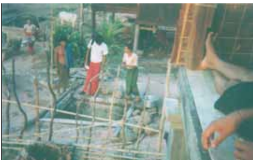
After BPHWT workshop villagers repair the well
