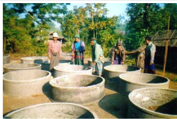
Constructing shallow-well water systems before installation - 2006
