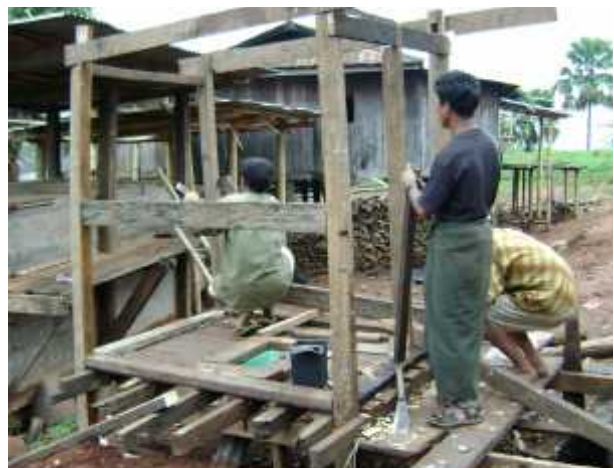
Building community latrines in Kavah- 2009
