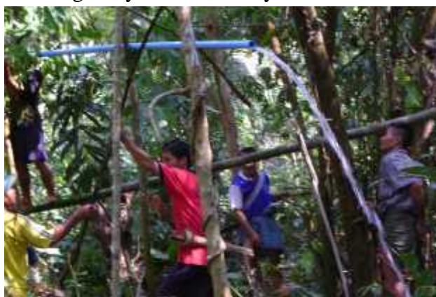
Building a gravity flow water system in Dooplaya -2009
