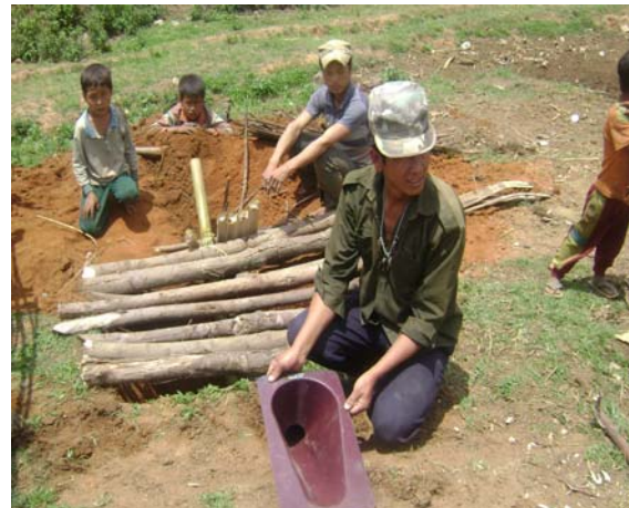
Building community latrines in Lahu area, 09
