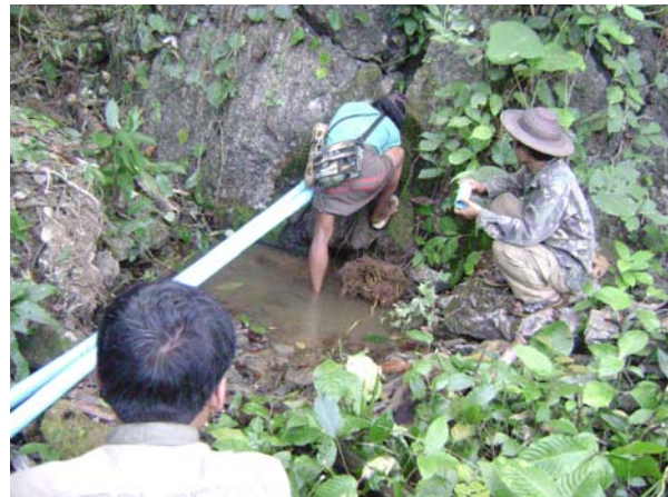
Gravity flow water system Pa An - 2009
