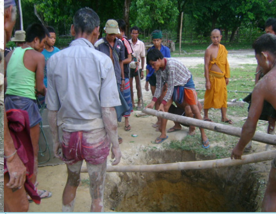
Building a latrine
