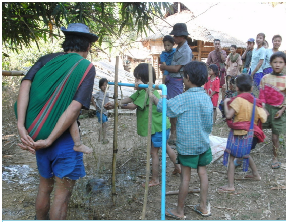
Installing a gravity flow water system
