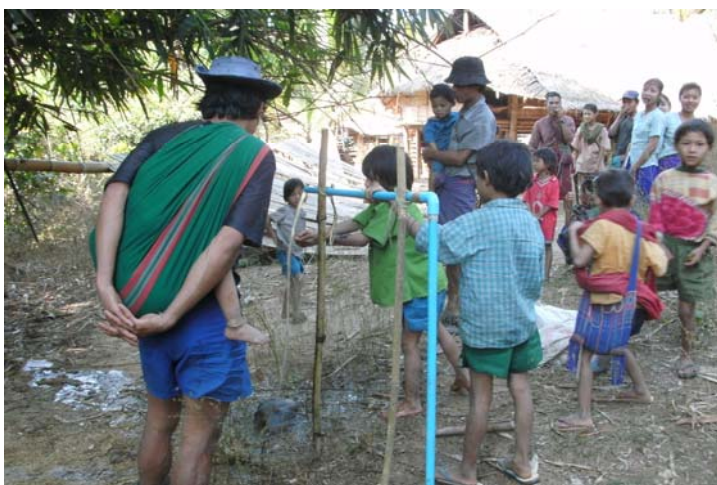
Providing a gravity flow to communities
