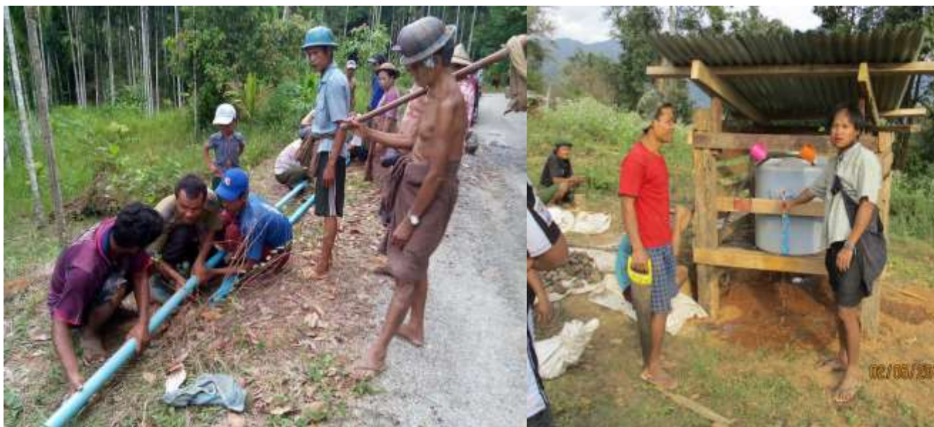
Installina water svstem in Yee and Taunao Field Area
