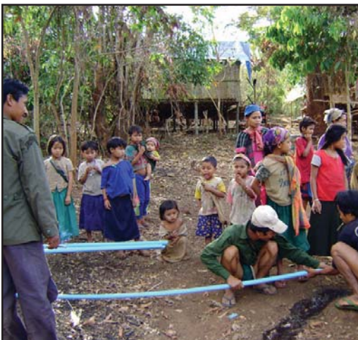
Assembling pipes to bring clean water to the village
