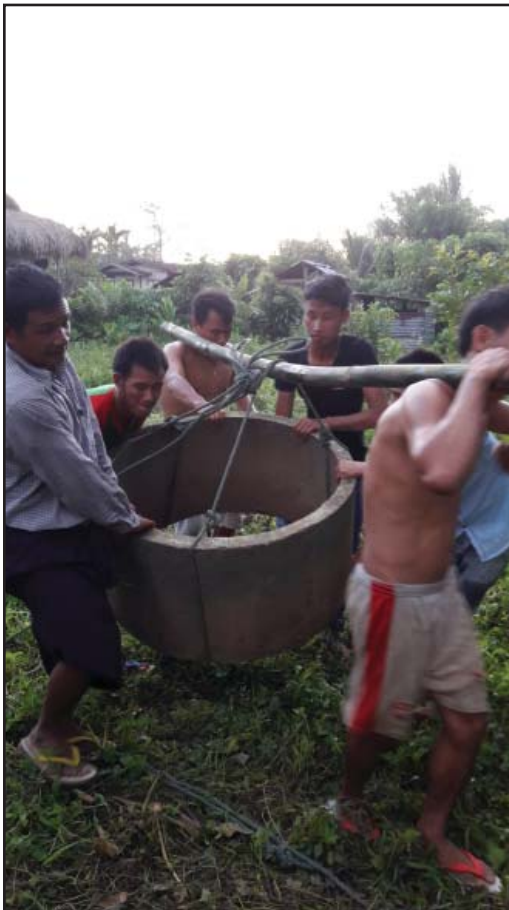
It is a group effort to carry the concrete cylinders used in constructing water storage!
