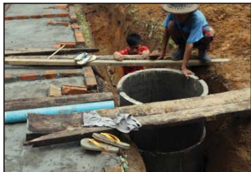
Concrete cylinders are placed to build the base of a latrine
