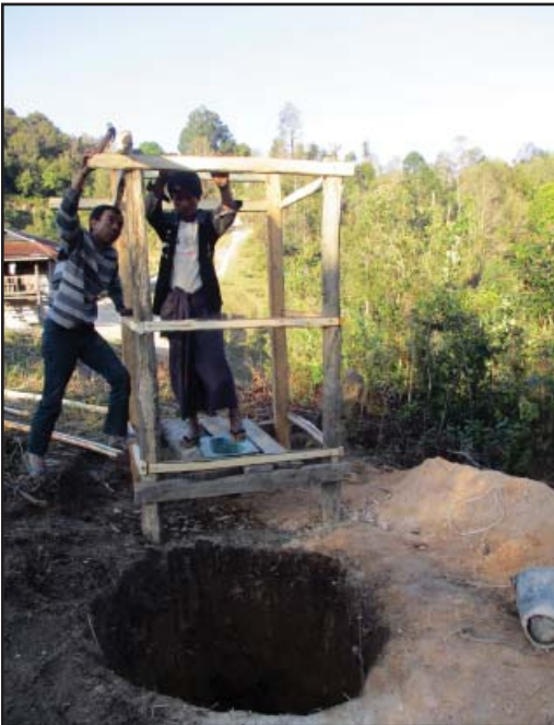
Framing is placed for a latrine
