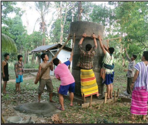
Villagers pitch in to build a concrete water storage
